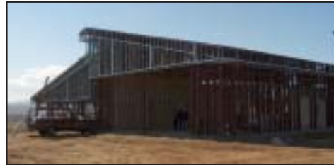
New Woodcrest Station Steel Frame
